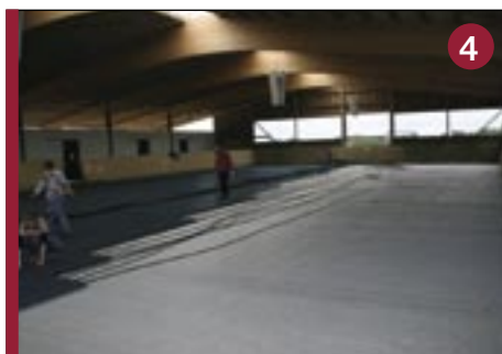
Installerar HIT-draingrid H55.0
