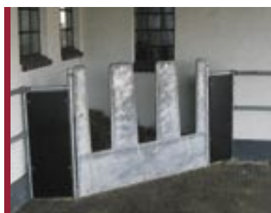
Installation at the edge of a building
